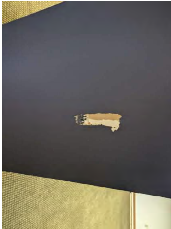
Photograph 4: Blue paint on drywall – no lead detected
