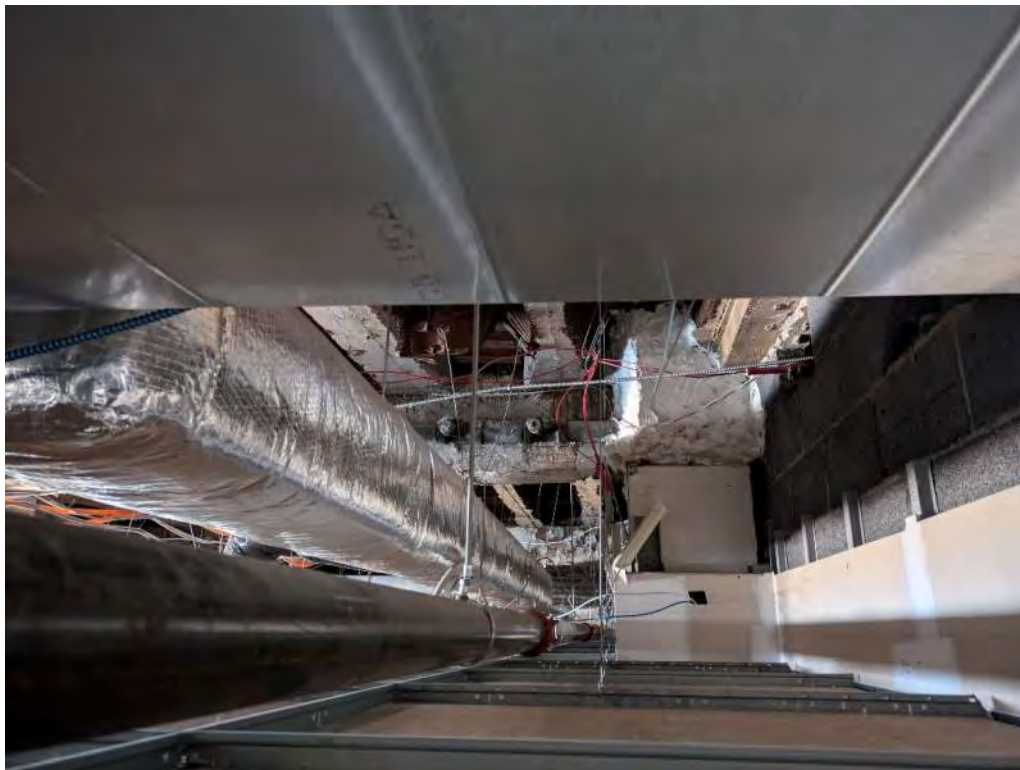
Photograph 11: Above ceiling on 14 th floor, East wing – plaster ceiling removed
