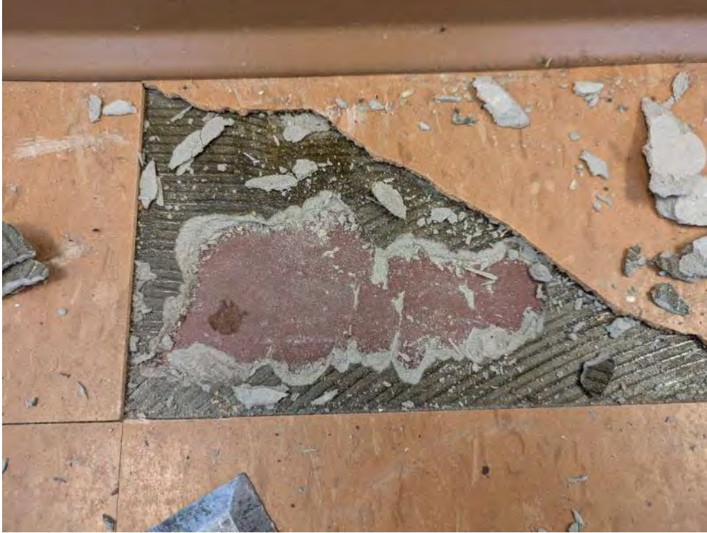
Photograph 13: Peach floor tile/glue (HA #7) – non-ACM, floor under is non-ACM floor leveler (HA #3)
